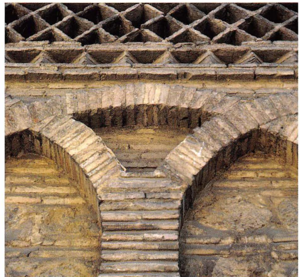
Intersecting arches at Bab Mardum Mosque, now called Church of Cristo de la Luz, were built between 998 and 1000 in Toledo, Spain.
